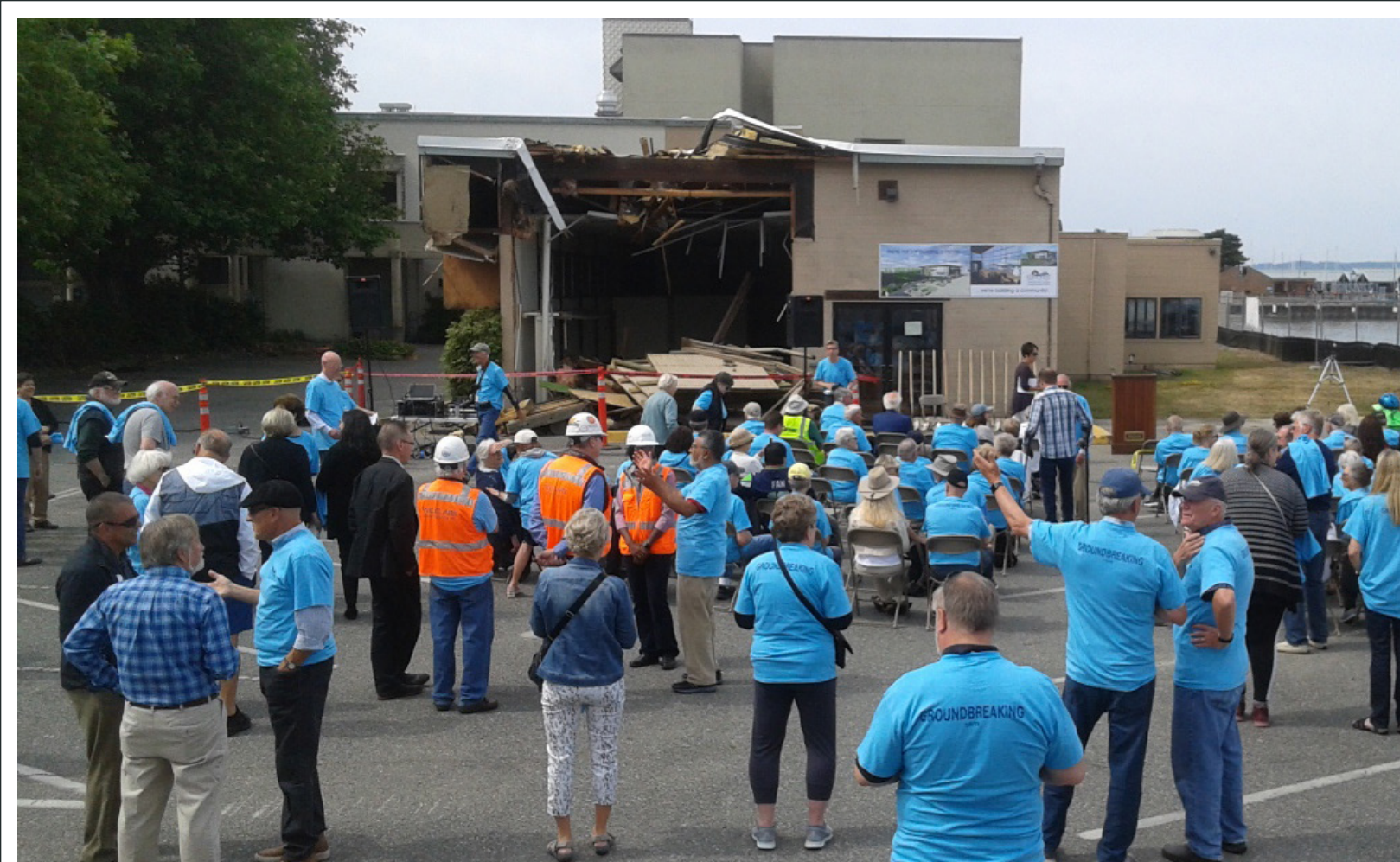
GROUNDBREAKING CEREMONY FOR THE NEW EDMONDS WATERFRONT CENTER (OLD SENIOR CENTER UNDER DEMOLITION IN BACKGROUND)
